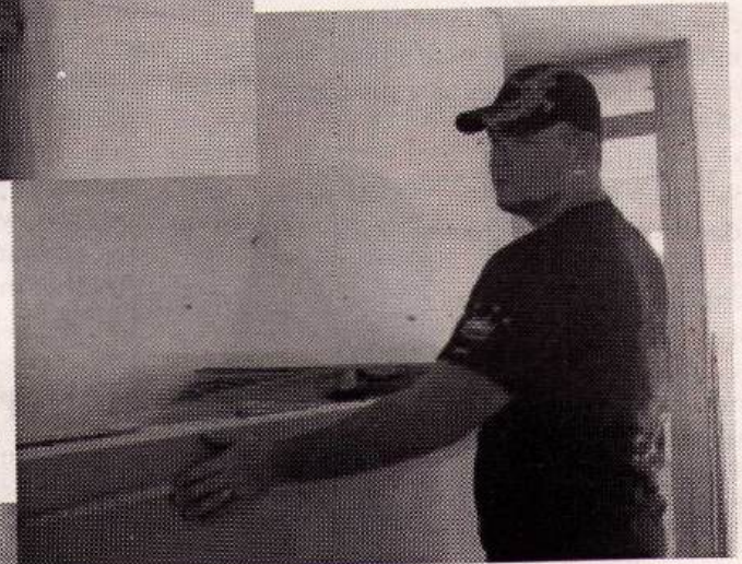
Mitchell James cuts a piece of drywall to fit on the wall of a coat closet off the living room.
