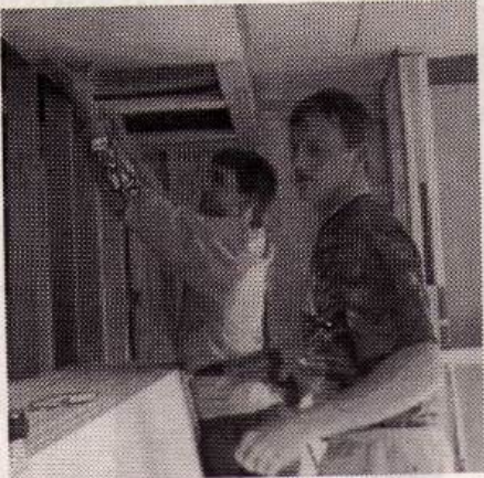
Seniors Joe Derby and Eric Steffes work on nailing drywall to the ceiling in the basement of the Building Trades house. The class is made up of 16 seniors from Marion and Linn-Mar.
