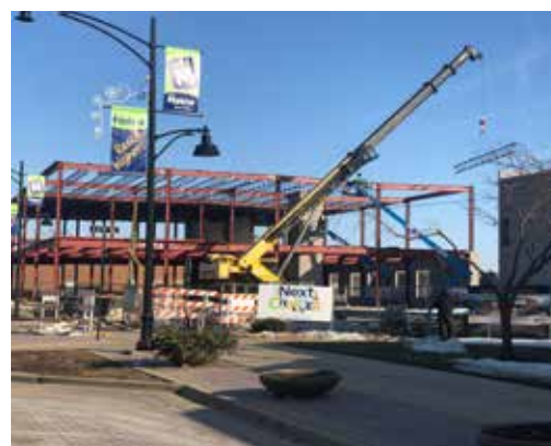
Construction continues on the “next chapter” of The Marion Public Library.
