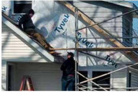
Two students work on the Flip House's roofing.
